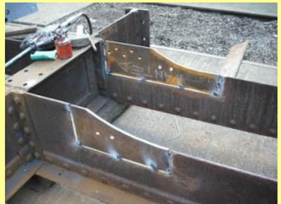
23/04/2011 - replacement of corroded sections of ladder frame.
