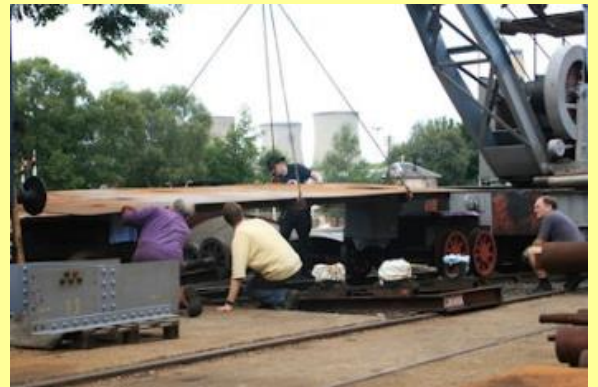
06/08/2011 - lifting the overturned tender base and placing it carefully on the accommodation bogies.
