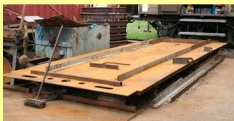
28/05/2011 - underside of the tender base plates
