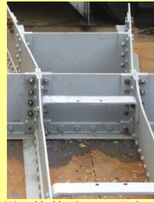
14/09/2011 - 'A' and ladder frames united and almost ready for riveting.
