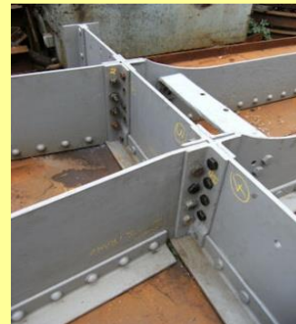
14/09/2011 bolts holding the 'A' and ladder frames in position.
