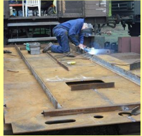
26/03/2011 - welding support angles on to base plate of new tender. The tender substructure is scheduled to be lifted and turned over in early April, so that work can continue.
