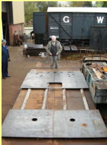
23/10/2010 - First pieces of the tender substructure steel laid on plinth.
