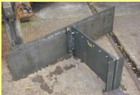
06/11/2010 - Steel work drilled for riveting. Spacer and one lead stringer, temporarily bolted together.
